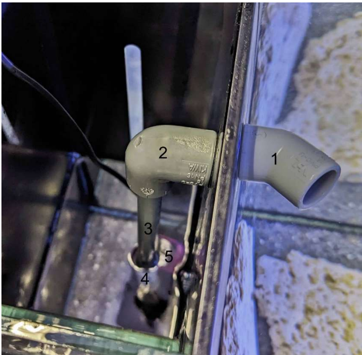
Fig. 4: Mounting the DC Runner 600
